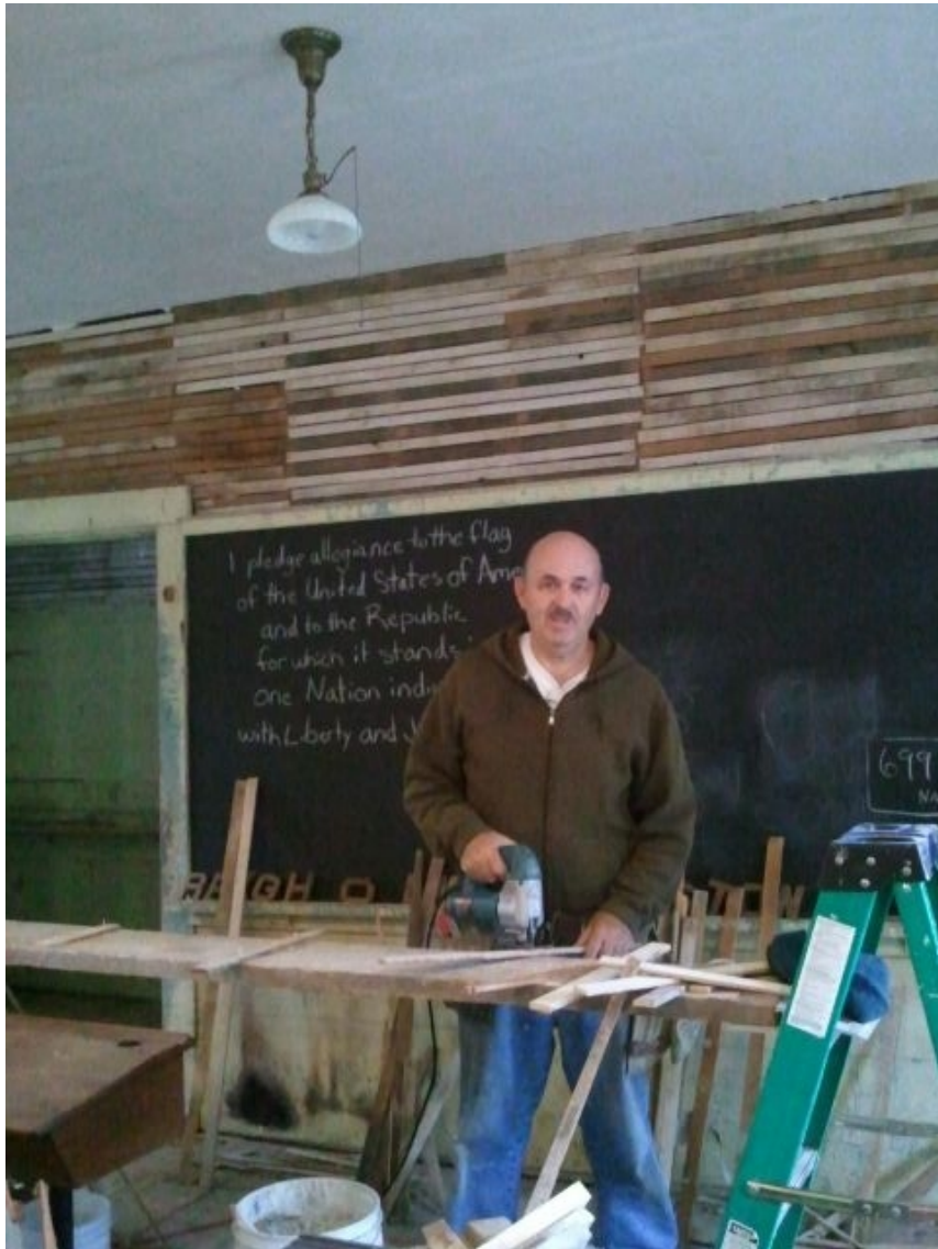
Ron Desrosiers installing lath at Holmes School
