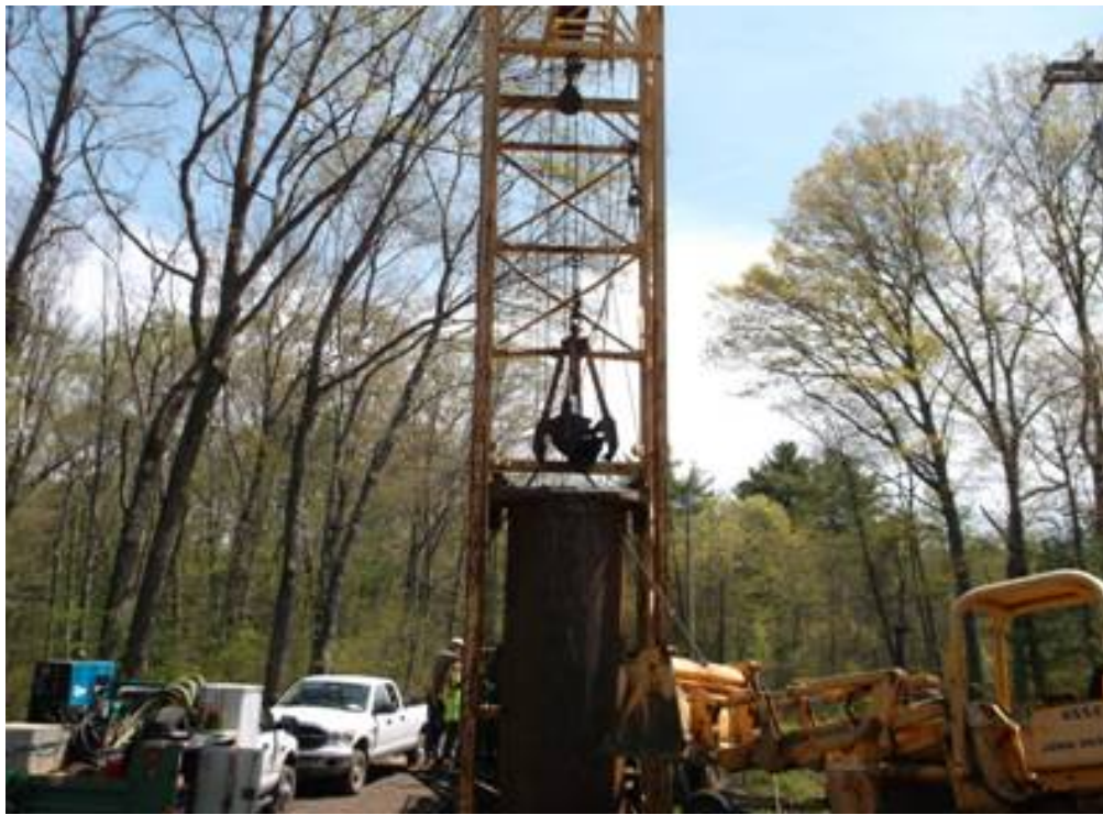
Installation of Well Casing Plainville 2 Satellite Well Project
