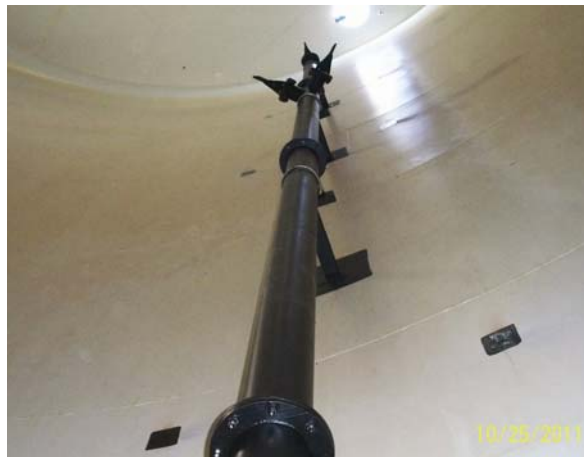
Hydrodynamic Mixing System in the Oldwood Water Storage Tank
